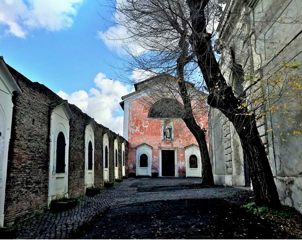
At the end of the Via di San Bonaventura, the Church's simple façade. The Stations of the Cross begin in the last stretch of the narrow street; the niches are visible on the left and on the façade of the Church
