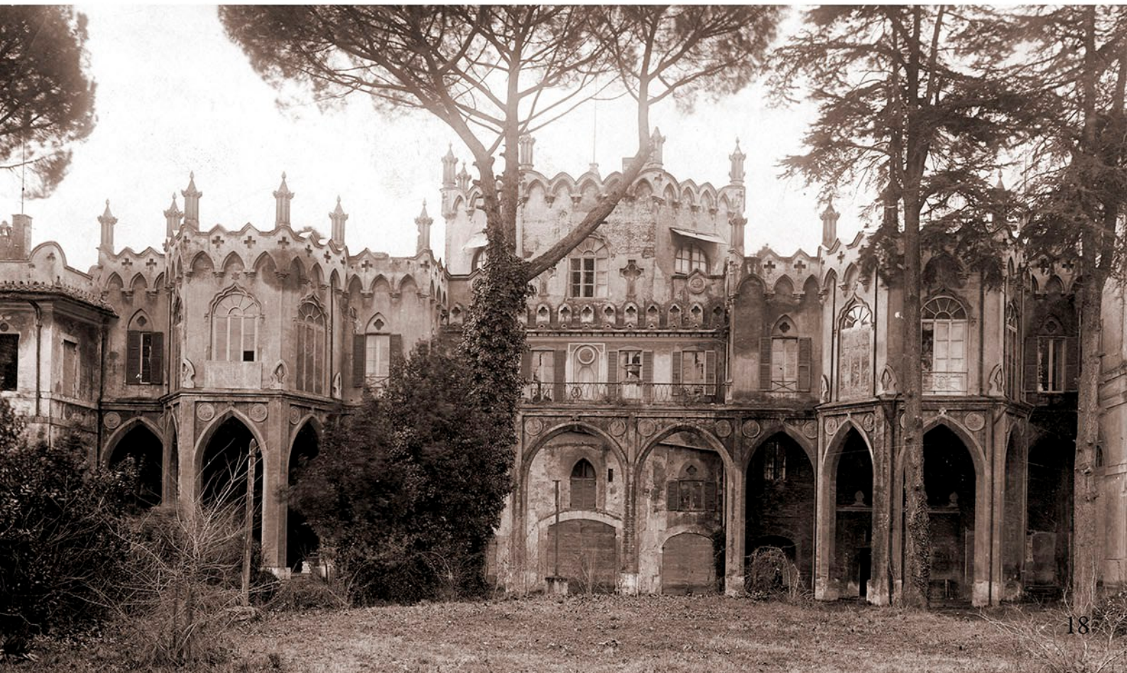
Villa Mills before its demolition
