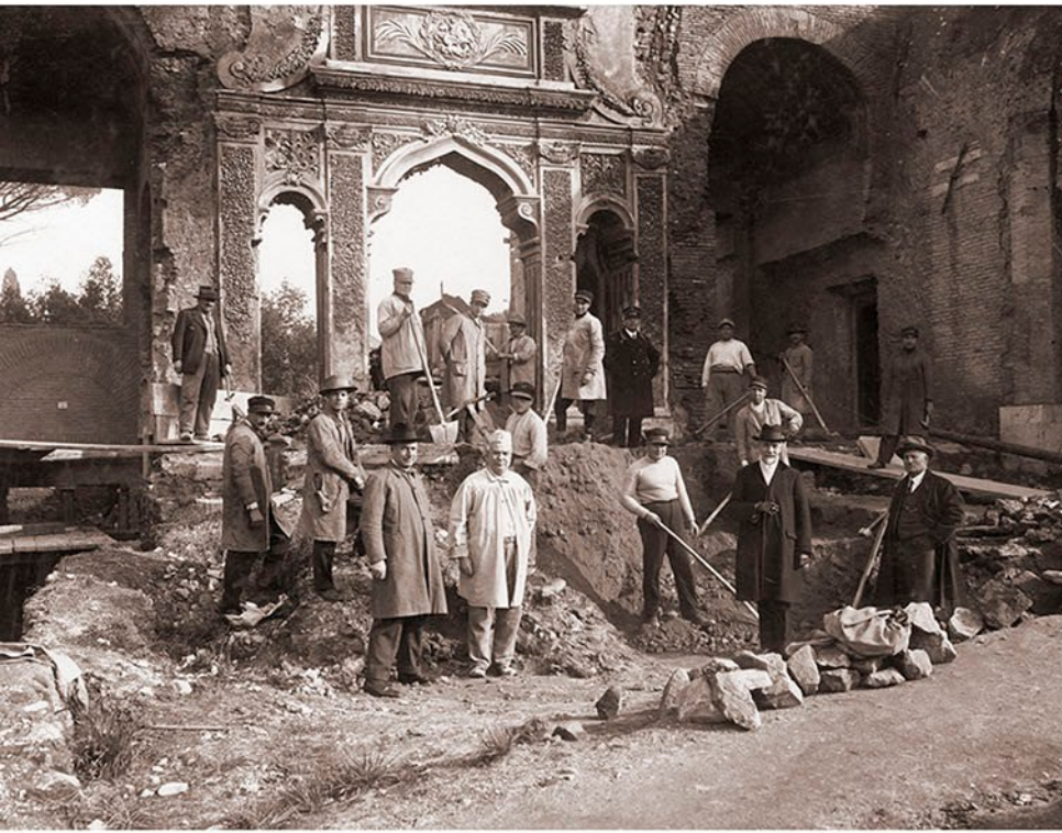
Villa Mills, demolition workers at work
