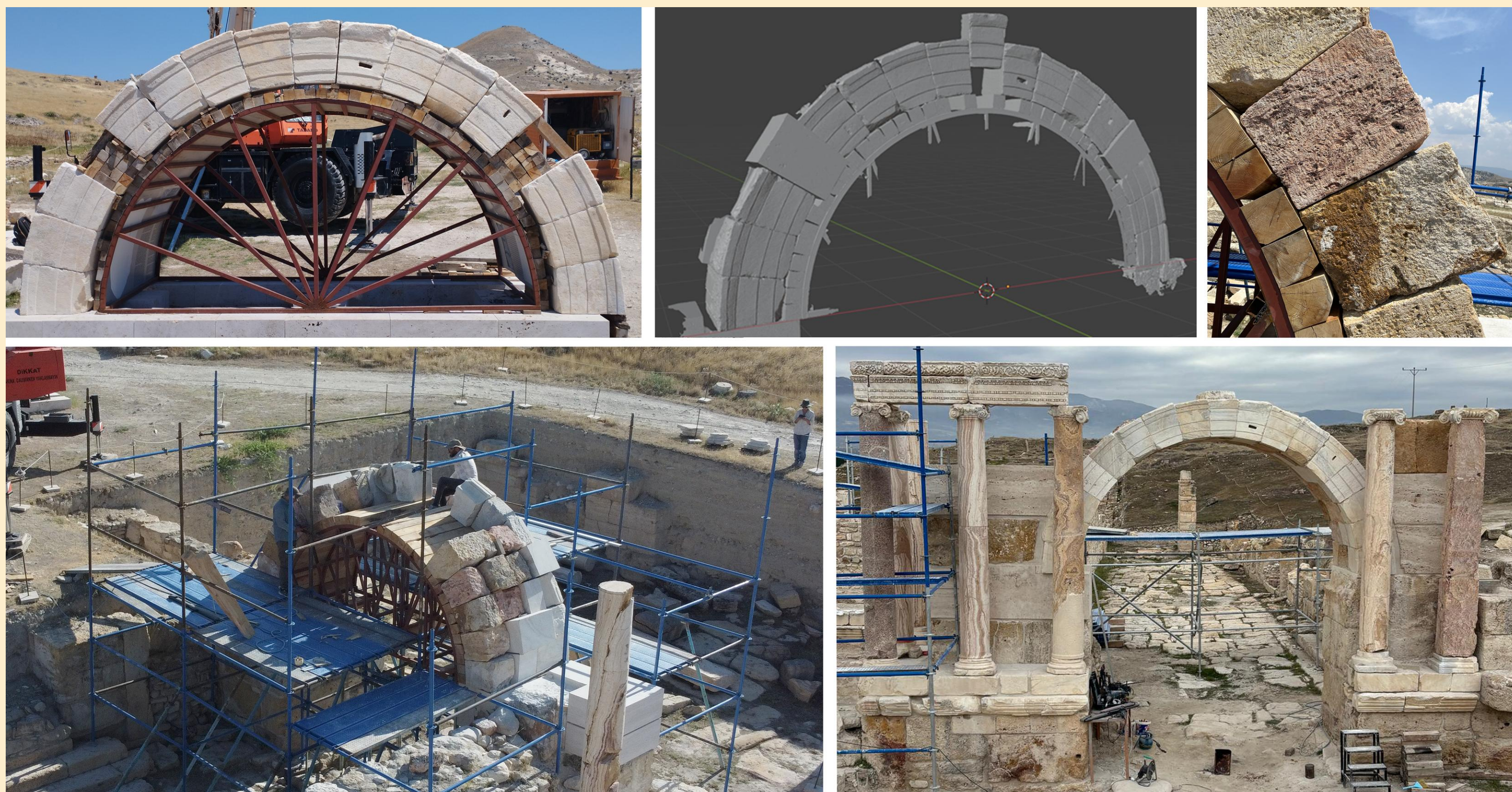
Fig. 4 The anastylosis of the vault on the north of the Nymphaeum (May-September 2025)
